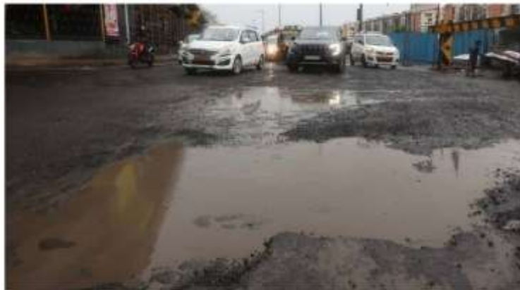
Ulwe road potholes near Sector 24 Navi Mumbai. (Express Photo by Narendra Vaskar)
