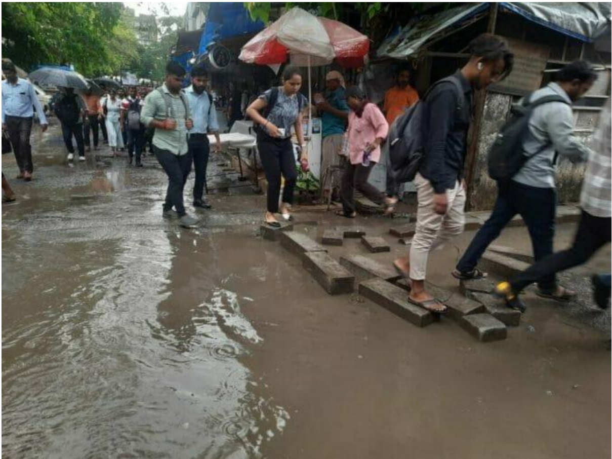
People find it difficult to walk due waterlogging outside the Kanjurmarg station. Pic: Stephin Thomas
